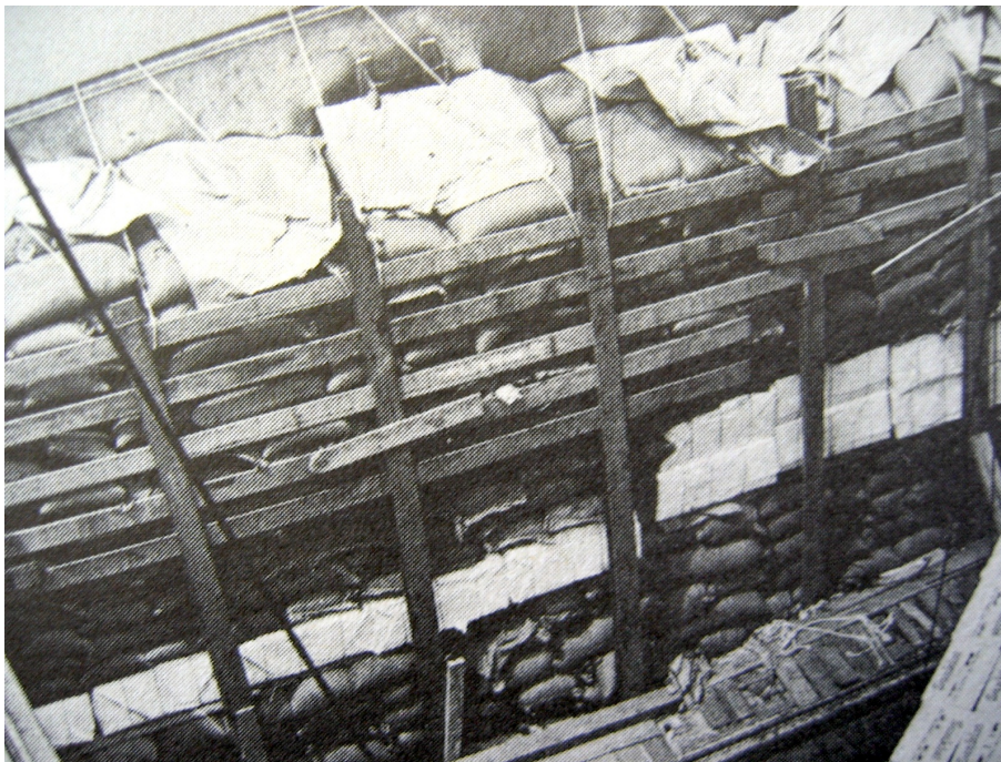
Figure 5: Dunnage walls (Source: Huntington, 1964:21)
