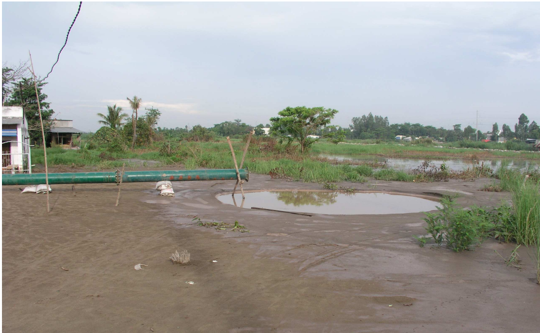
Figure 67 Levelling up land for development
