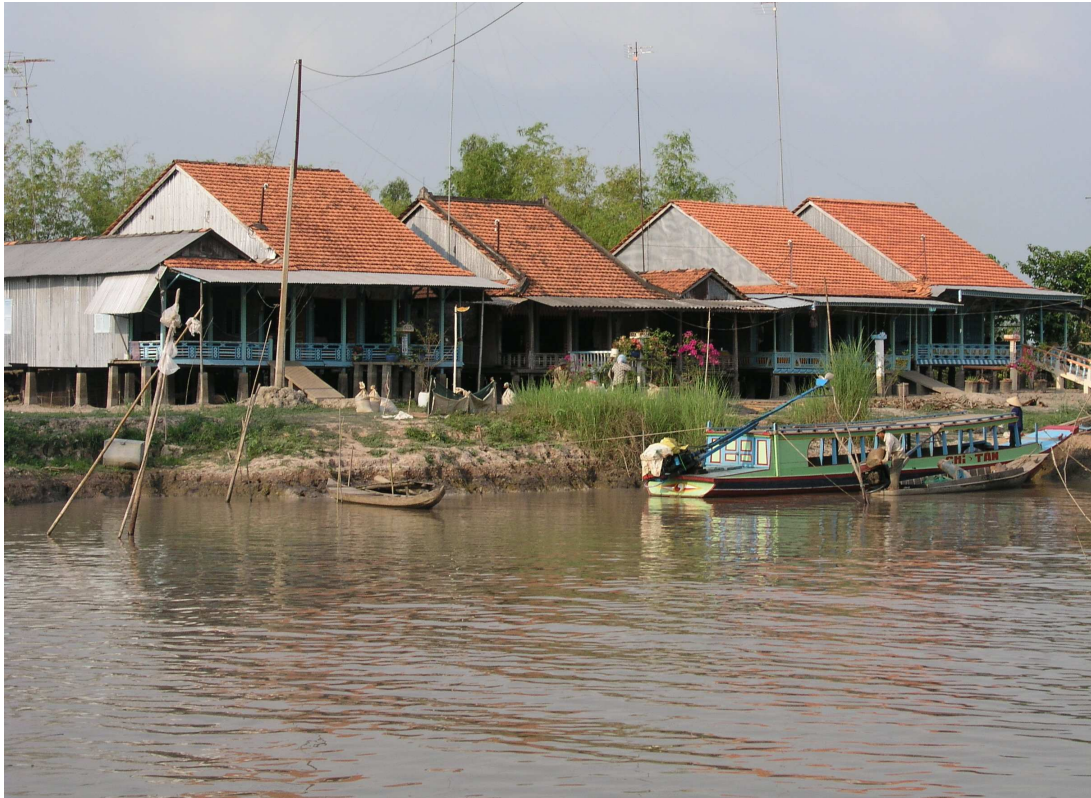
Figure 3 Houses in Vinh Binh Commune raised on stilts beside the river
