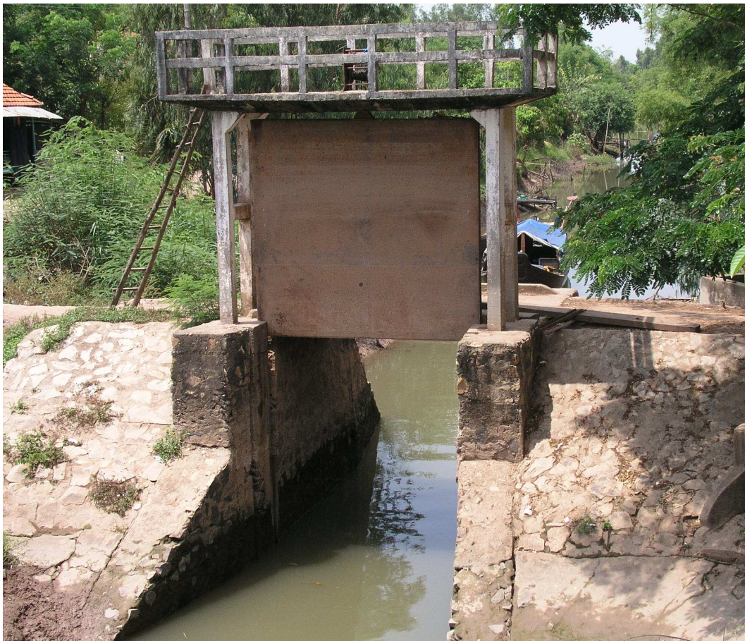
Figure 42 Sluice gate set into a high dike
