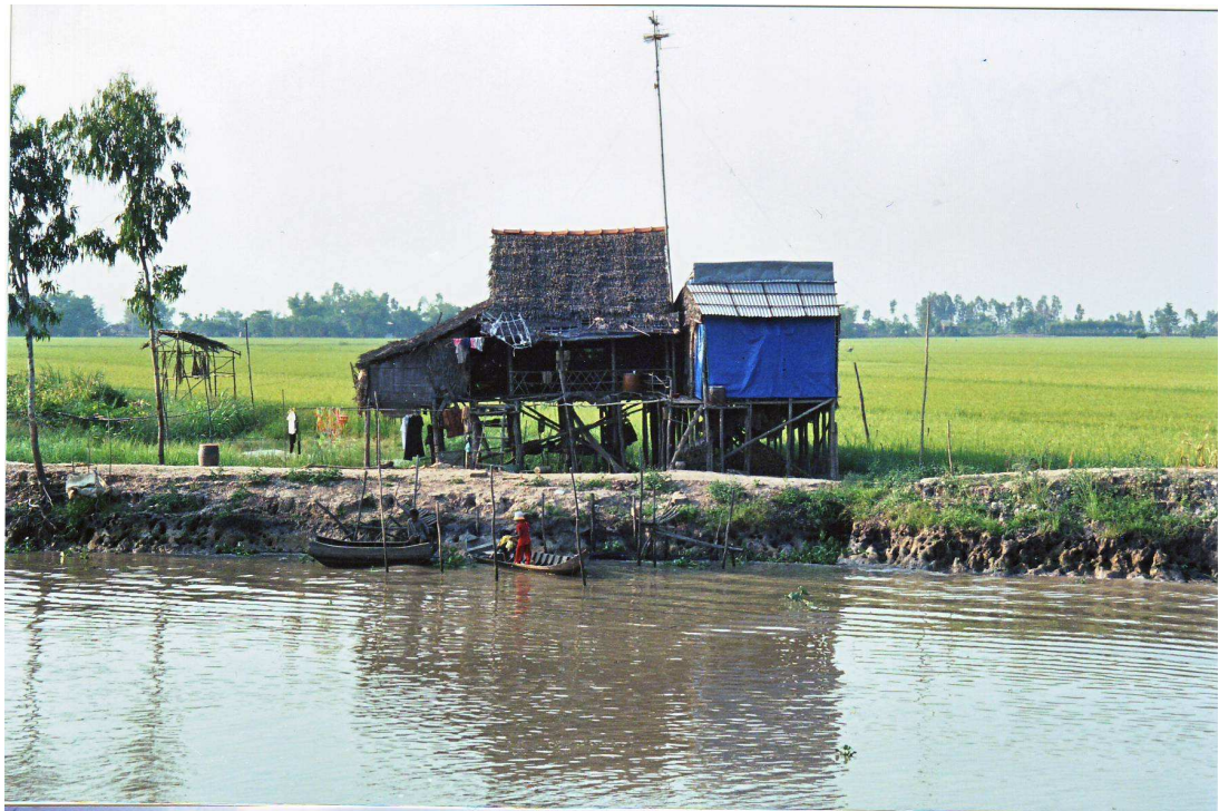
Figure 30 House located on stilts on an August dike
